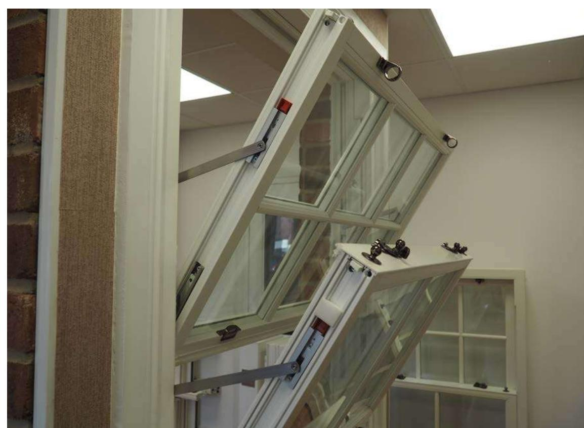
\* PLEASE NOTE DO NOT SLIDE WINDOWS UP WHEN IN TILT POSITION ON SPRAYED WINDOWS AS THIS CAN SCRATCH AWAY AT PAINT. ONLY USE ON SPRAYED WINDOWS FOR CLEANING NOT EVERYDAY USE.
