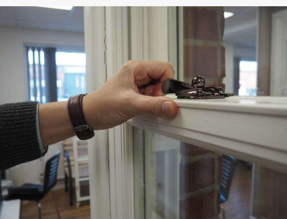
To close and lock, close both sashes by reversing the procedures above, then close the lock by turning the lever clockwise. Finally, lock the window with the key supplied.
