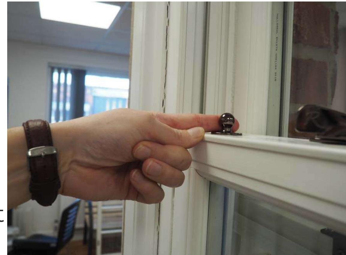
Next, completely lower the top sash using the ring pull handles.
