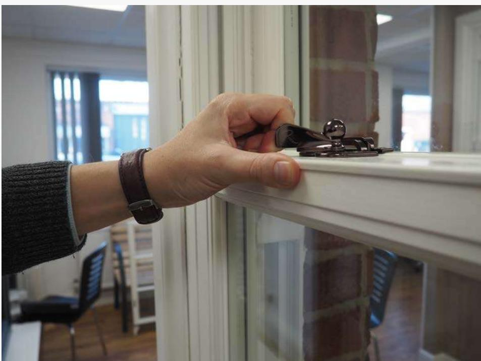
Operating your sash windows is extremely simple. Just unlock the window and then slide the bottom sash up and/or the top sash down as required.
