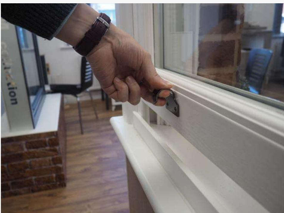
Unlock the cam catch(es) with the key supplied, and turn the lever(s) anti-clockwise to open.
