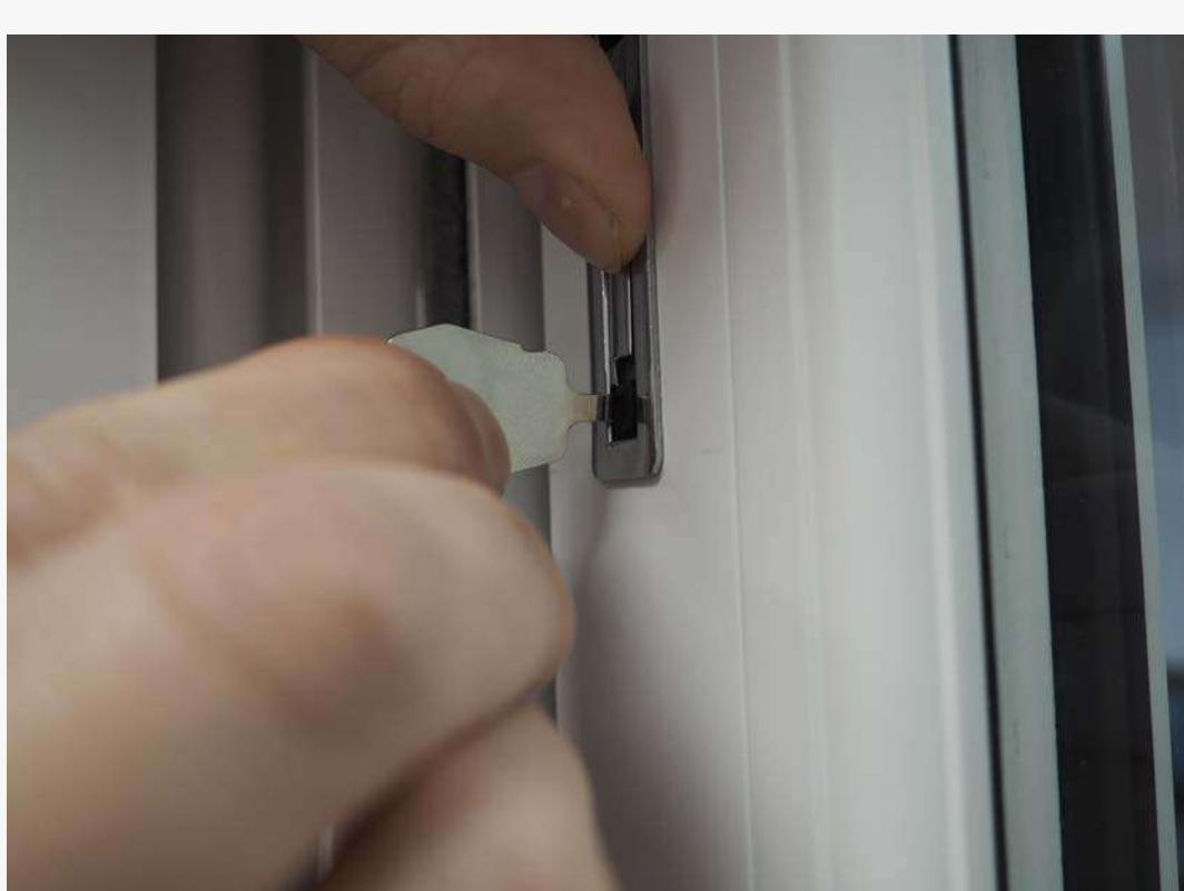
With one hand push and hold the limit stop in, and then with the other hand turn the key.
